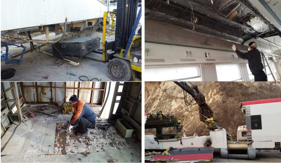
Fig. 1. Pretreatment and dismantling steps of ELRS (One of the authors took the photos)
